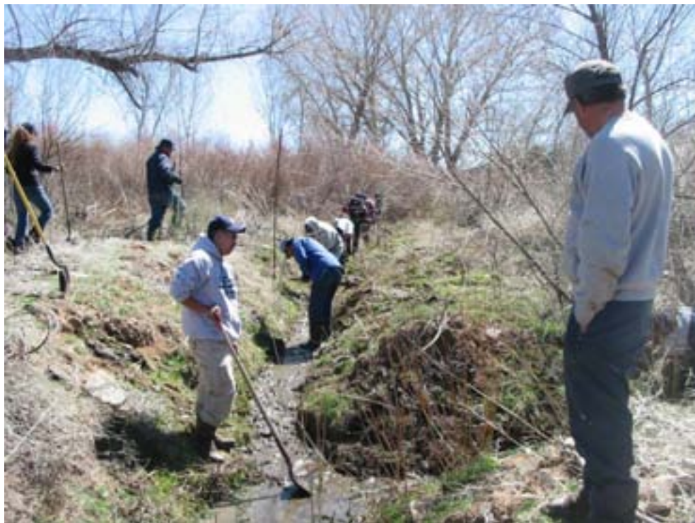
Figure 6. Cleaning of the Acequia
